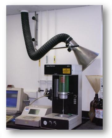
laboratory technicians were disposing of excess test samples, pouring the samples into the funnel and which drained into the drum. This horseshoe shaped vent captures the fumes and odors released from these samples. The New-Tech<sup>™</sup> horseshoe **Spot Exhauster** is fabricated with a built in swivel joint at the connection from the neck to the horseshoe perforated pinpoint exhaust vent, allowing easy replacement of the drum.
